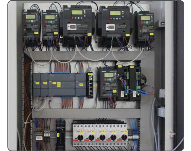
PLC KONTROLLÜ ELEKTRİK PANOSU PLC CONTROLLED ELECTRIC PANEL
